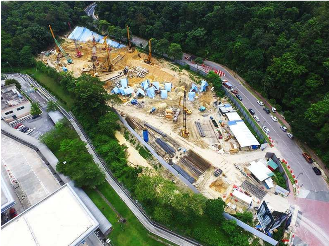
Aerial View of Construction Site
