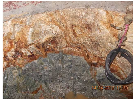
Caisson Rock Socket
