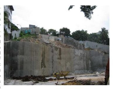
and the disturbance has been successfully reduced to the minimum. We can concur that hand-dug caisson is an ideal solution when come to the hill slope development.
