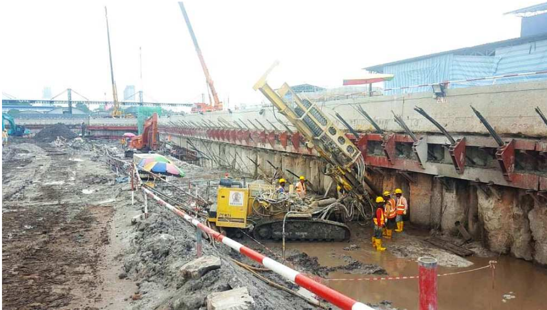
Photo 1 : G-Klem Machine is carrying out the drilling work
