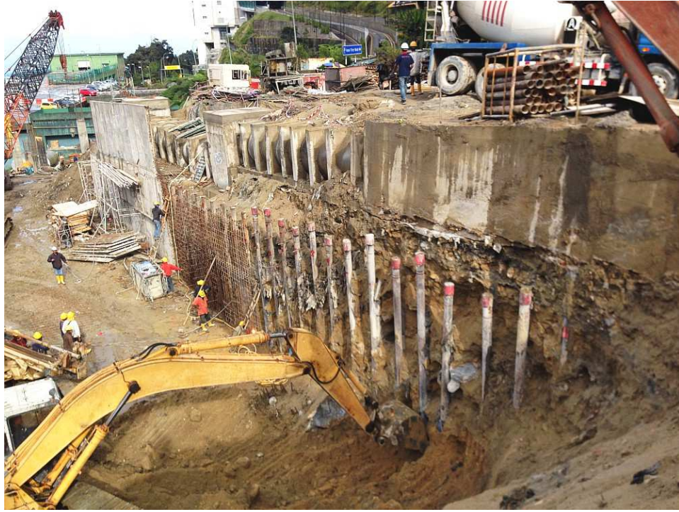
Wall in Construction
