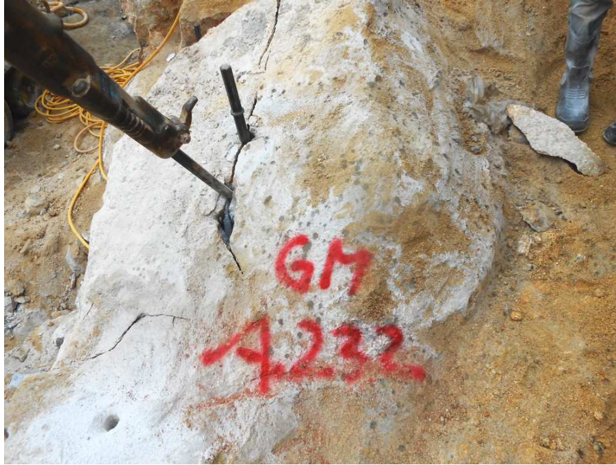
Figure 5 : Rock Splitting at Genting Mall
