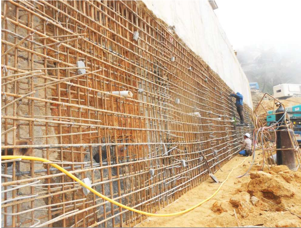
Figure 2: Construction of Skin Wall and Soil Nail Bearing Plate Installation.
