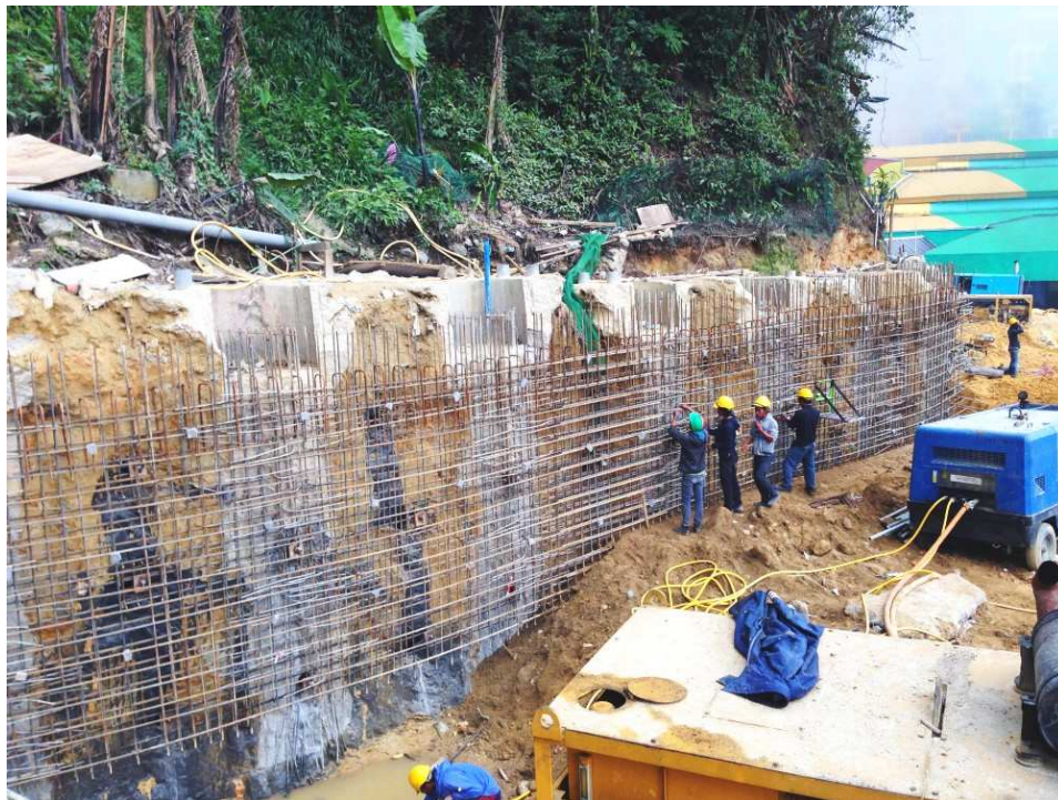
Figure 1: Fabrication of R.C.Skin Wall after the Earthwork Excavation in Stages.
