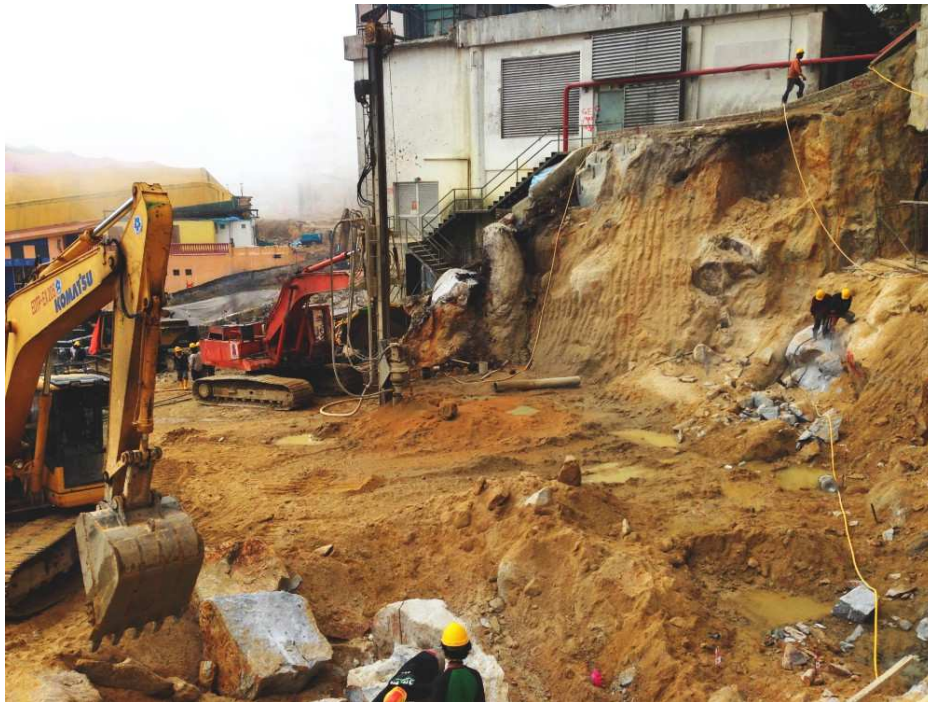
Figure 6 : Rock Hacking at Genting Mall
