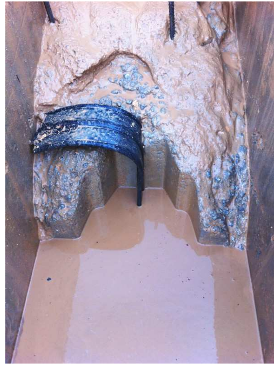
Profile of construction joint with centre bulb rubber water stop
