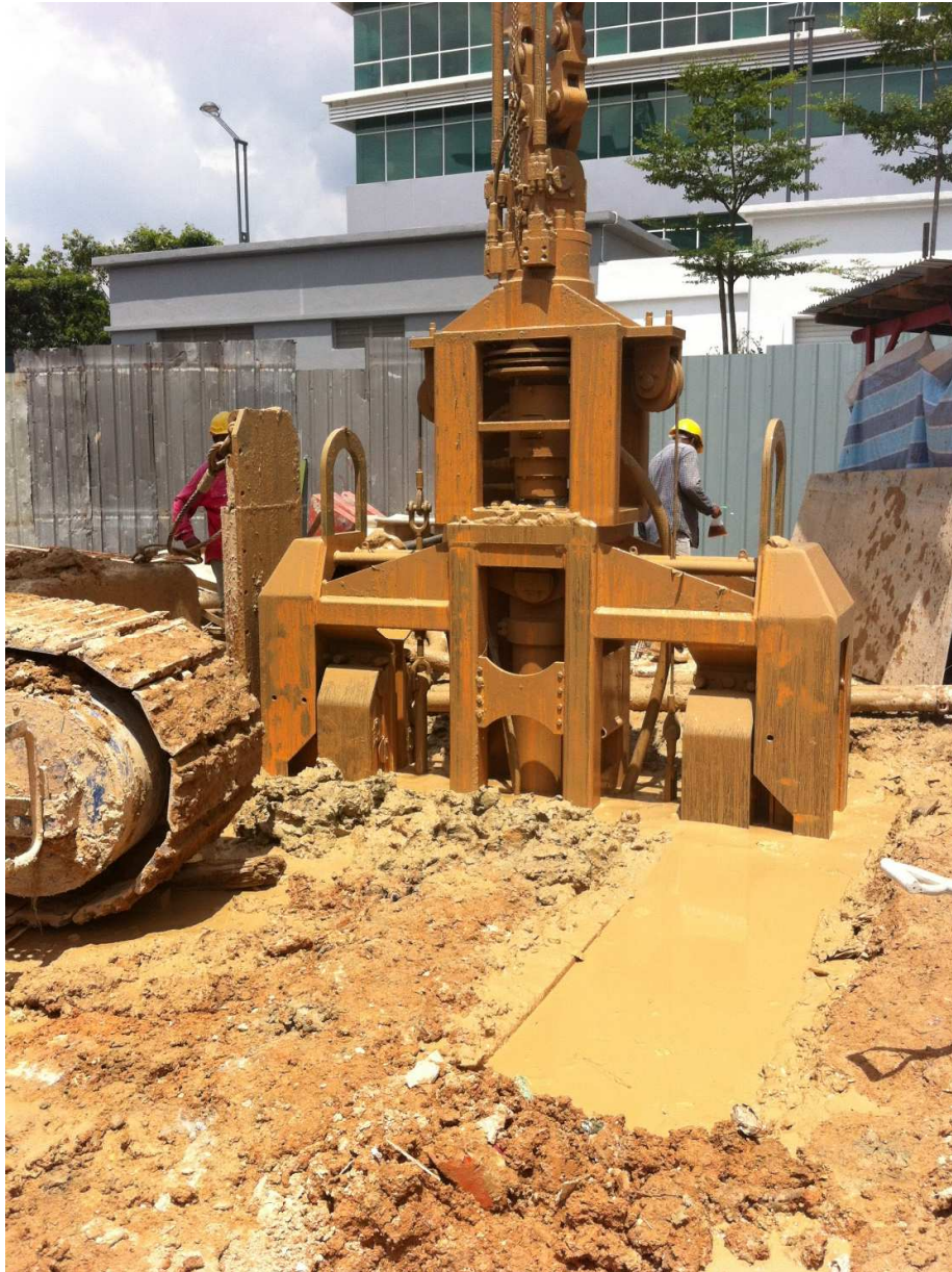
Excavation of corner panel
