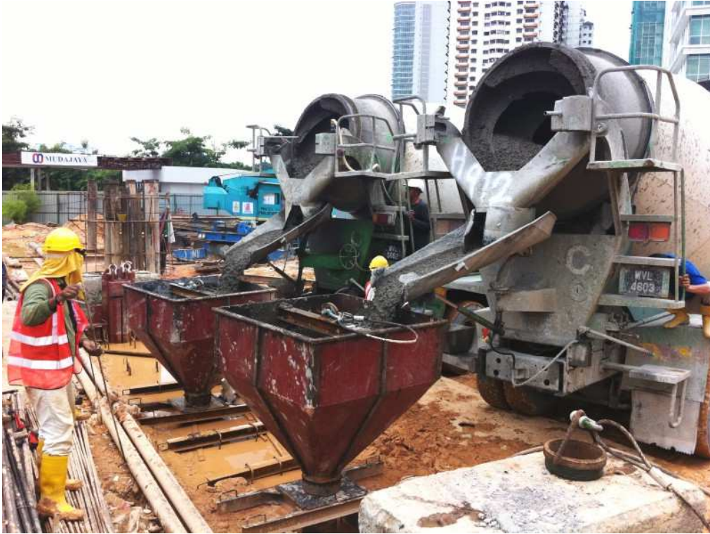
Concreting of wall panel
