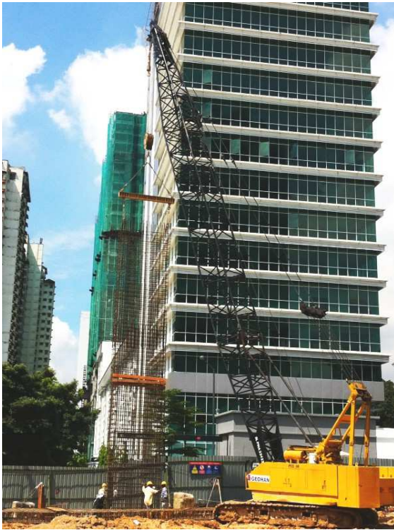
Lowering reinforcement
