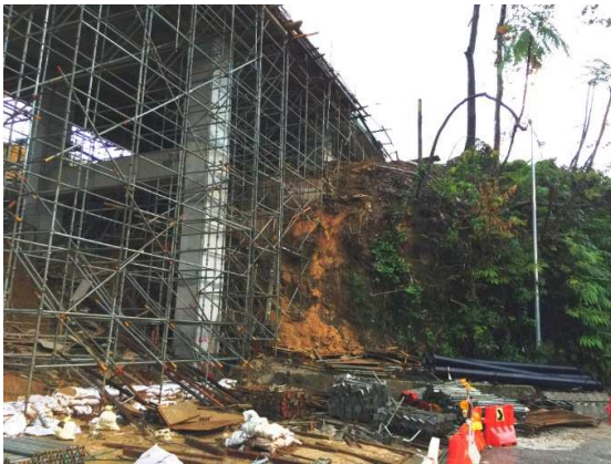
RC Deck 2 Construction on Valley
