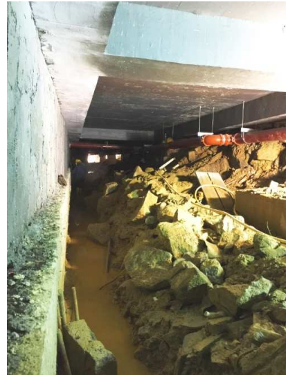
Massive Manual Rock Hacking
