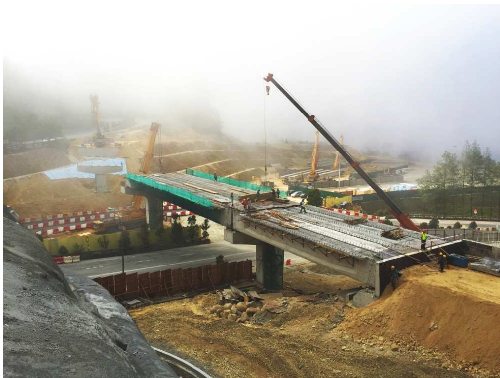
T-Beam Launching Progress Photo
