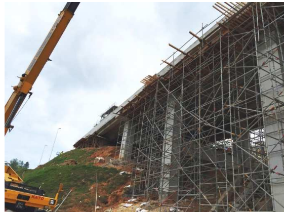
RC Deck 2 Construction on Valley
