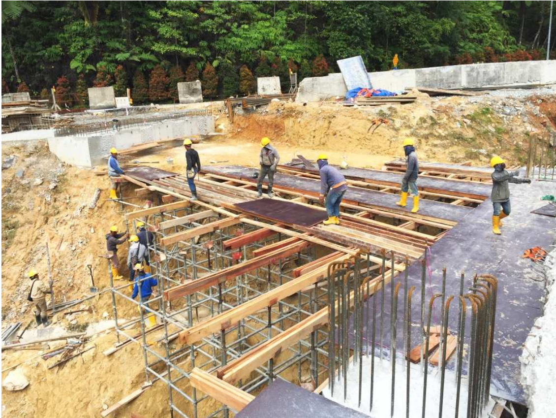
Bridge 2 Construction on Slope Terrain
