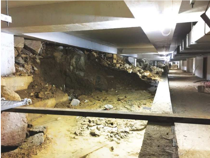
High Bedrock Level along RC Drain Alignment
