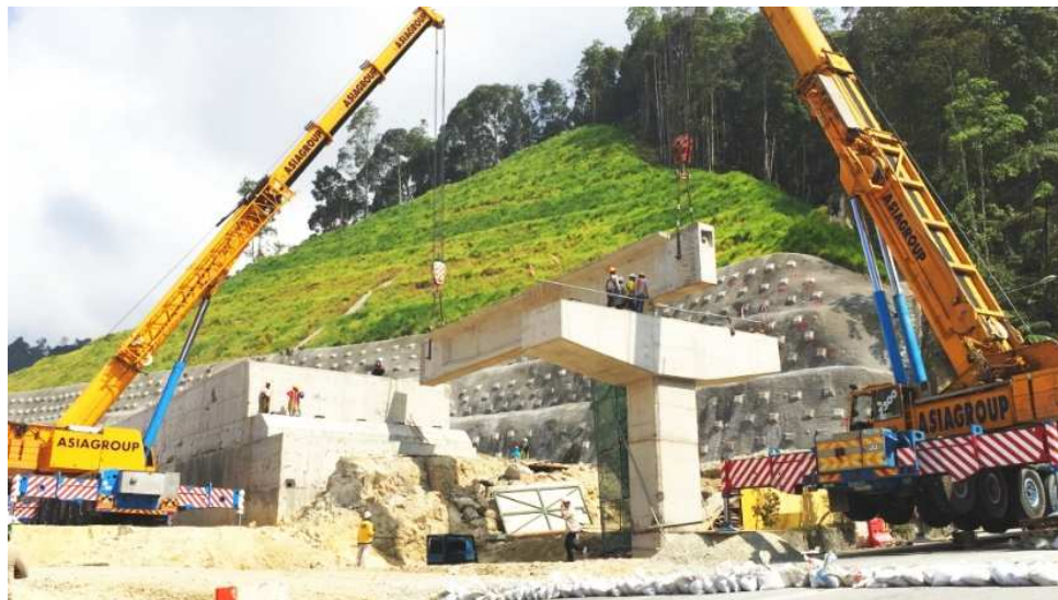
T-Beam Launching from Abut A to Pier 1
