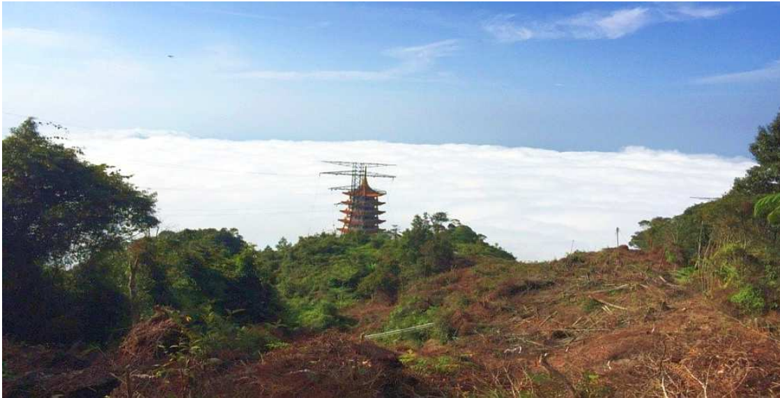
Photo taken during construction stage
