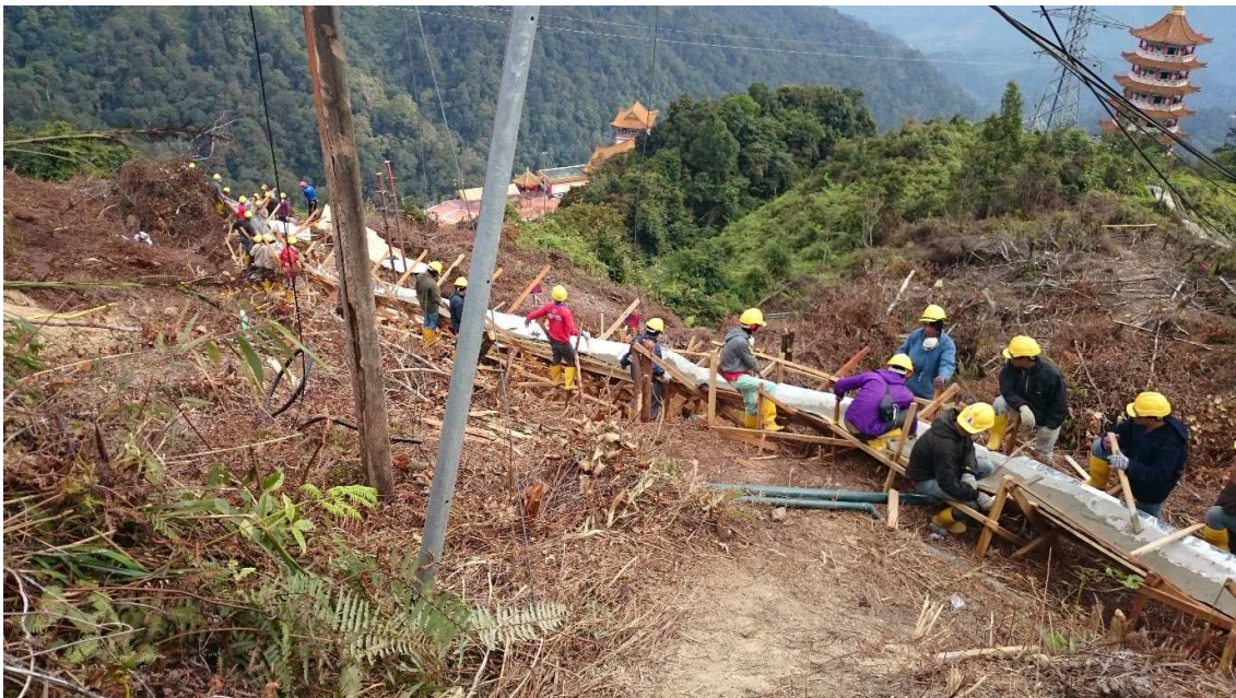
Temporary Concrete Chute
