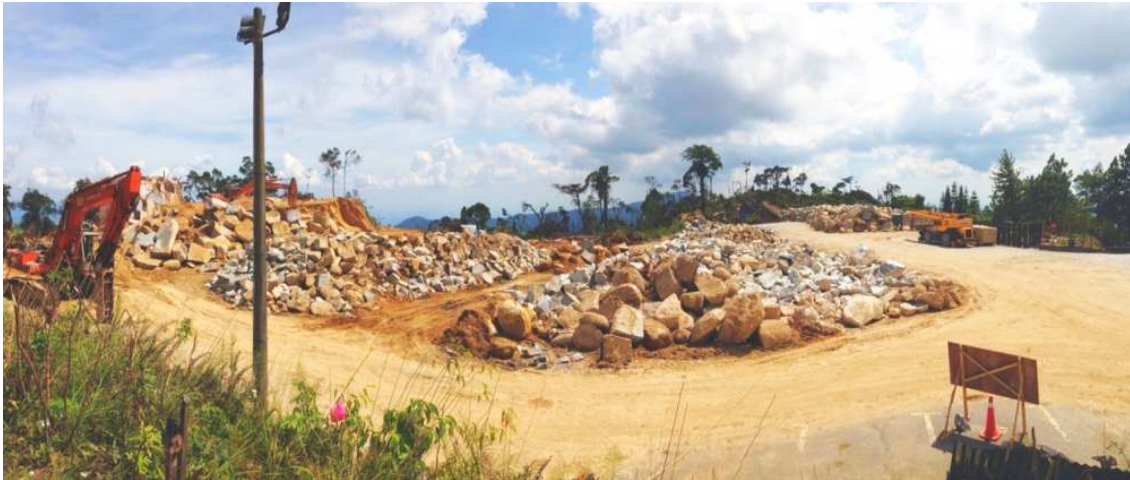
Plant and machineries were deployed to break down the boulders into smaller fragments before they were practicable to be transported out to designated dump site.
