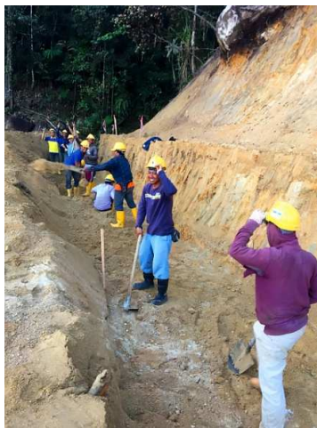
Excavation of Trench
