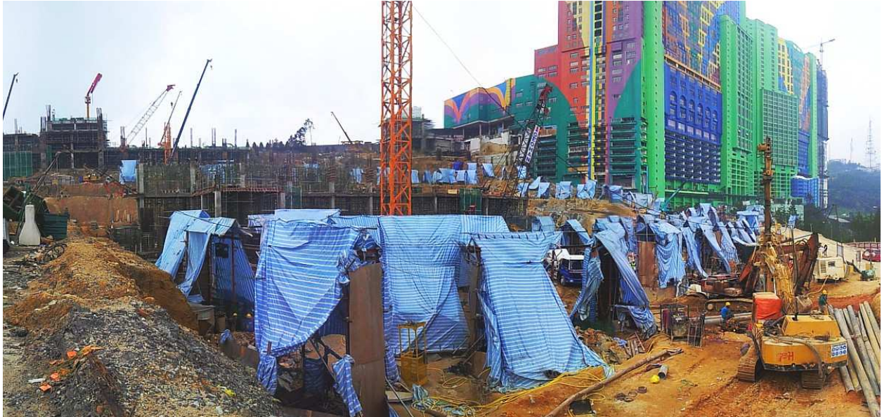
Tower 3 & 4 Site Photo
