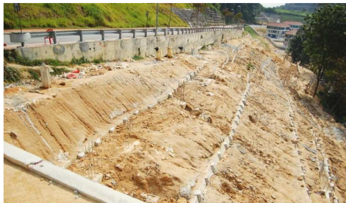
Completed Micropile Works
