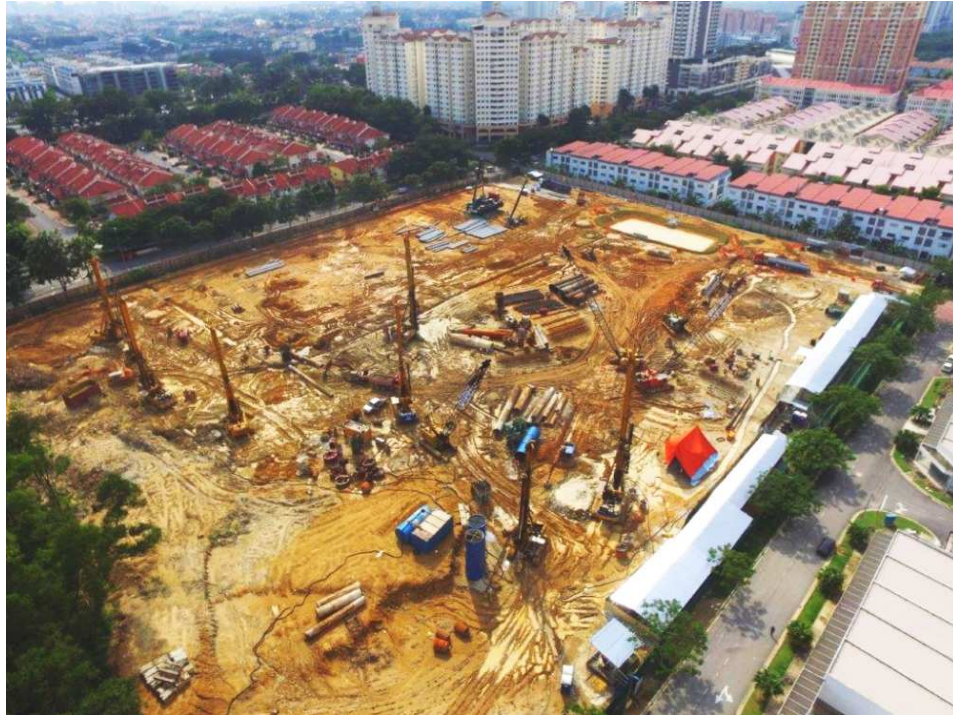
Aerial View at Site during Construction Stage
