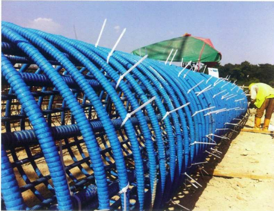
GFRP Reinforcement Cages of 1200mm Diameter, "Soft Eye" piles; Main Bar: 25mm; Spiral Links: 20mm (fabricated in spiral coils from factory)
