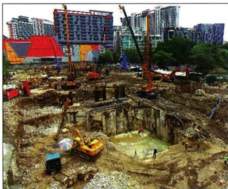
Figure 7 – Deep Excavation of Liftcore
