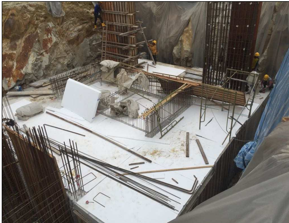
Figure 7 : Insulation Done on Footing LC3
