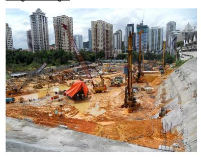
Based the subsurface investigation report, (SI) geological profile of the site is granite residual formation with varies of bedrock level and inconsistency of weathering grade of Granite rock over the site. The pile is designed to be founded on rock socket or maximum fixed pile length if no rock was encountered. Due to the deep layer of overburden soil, the soil friction is taken into account for optimisation of rock socket length required.
